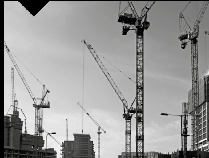
CONSTRUCTION WORK AT NINE ELMS
